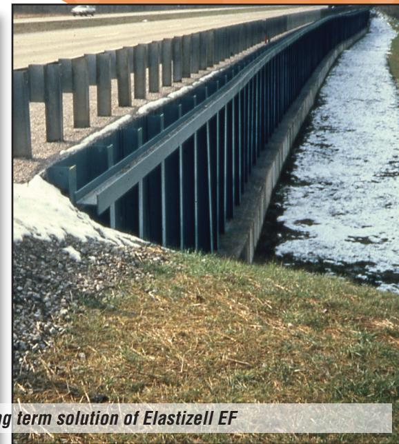
*Portion of slip material excavated and replaced with lighter long term solution of Elastizell EF*
